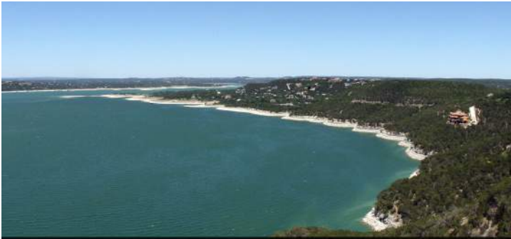
The 2 mile (3.2 km) long, 9-foot (2.7 m) diameter raw water tunnel carries water from Lake Travis to the Austin WTP4 treatment plant, through the raw water pump station. An additional 6.5 miles (10.4 km) of finished water tunnel distributes water from the plant to the citizens of Northwest Austin and Travis County.
