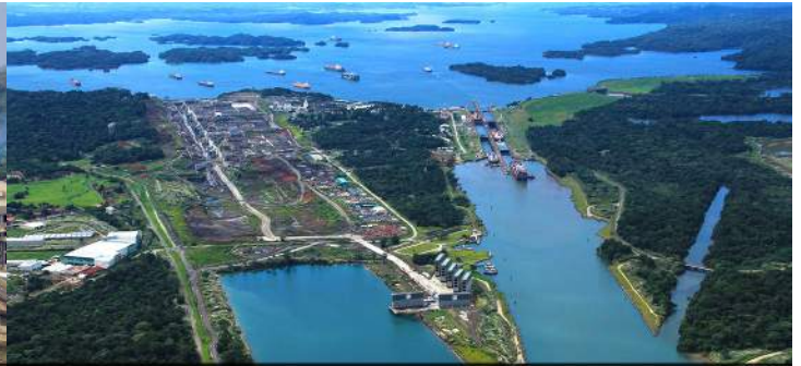
The new Atlantic Locks Complex is adjacent to the existing Gatun locks.
