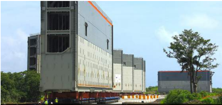
Lock Gates - the largest in the world - weigh in at an average of 3,100 metric tons each and operate by rolling across the entire lock lane. The MWH-led team designed 16 rolling gates - eight each for the Atlantic and Pacific locks.
