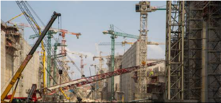
Navigation Locks - each chamber is 426.72 m (1,400 ft) in length - nearly as long as the Empire State Building is tall. There are three lock chambers on the Atlantic side and three on the Pacific side.
