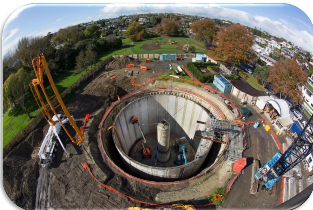
Figure 22: Overall site view during construction with GRP liner in tank center
