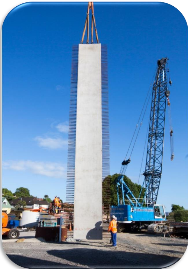
Figure 20: Precast wall panel and crane lift pad
