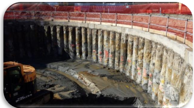
Figure 19: Tank excavation showing soil columns on perimeter
