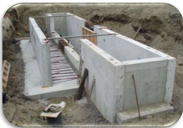
Figure 12: CSO Chamber under construction
