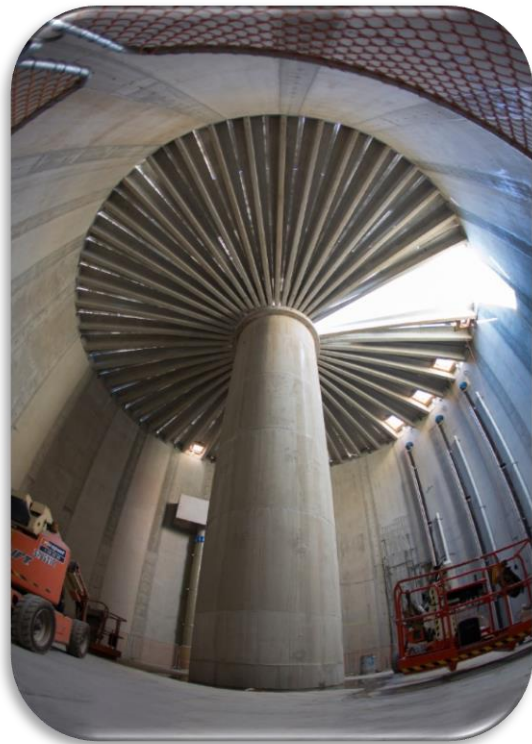
Figure 13: Tank Centre Column Showing PC Wall Panels and Roof Beams
