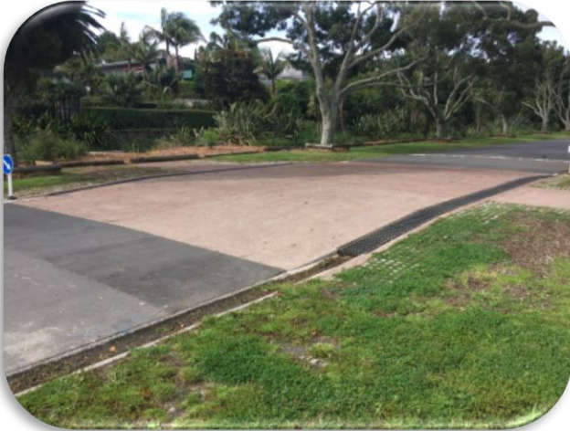
Figure 8: Completed speed table to protect pipes and allow bus access
