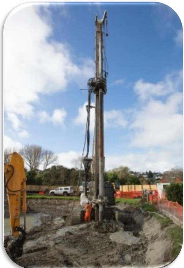
Figure 18: Site Works Commence with Installation of DSM Columns
