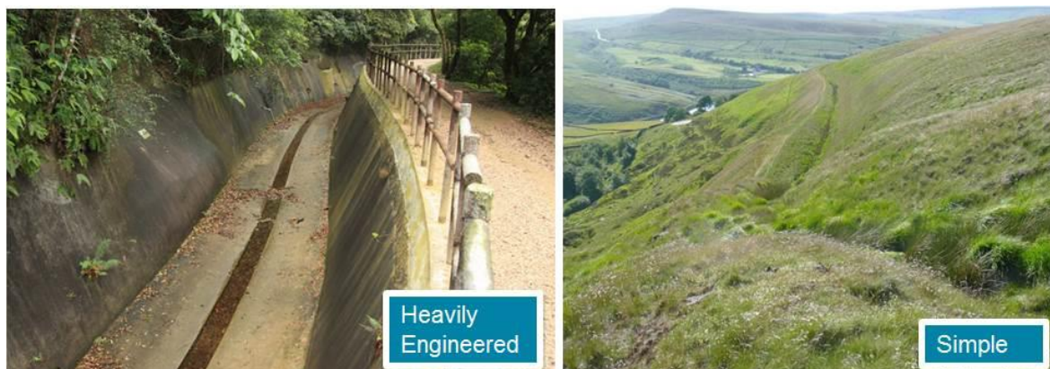
Figure 2: Source control – Catchwater diversion channels
