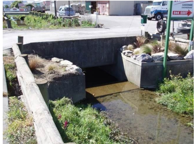
Photographs 5 & 6: Beach Road Drain during a high tide (left) one of the constricted bridges (right)
