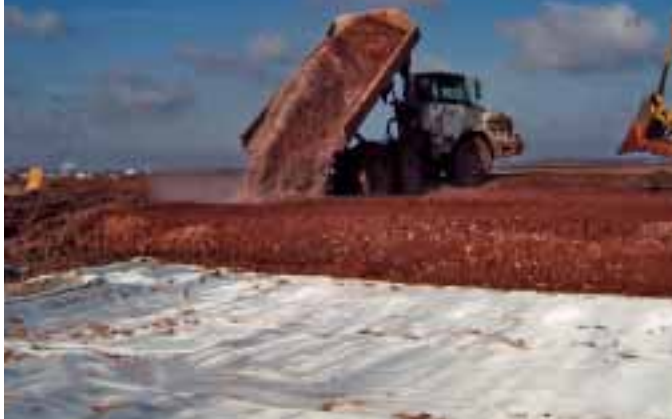
Dewatered tailing materials from Balen are trucked to disposal areas
