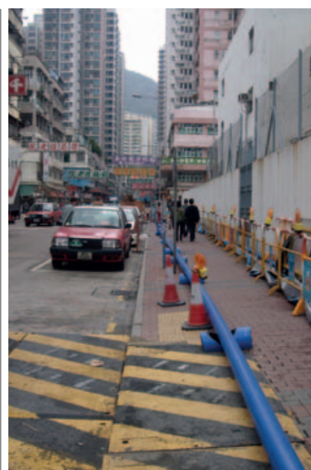
The US company Insituform completed a polyethylene lining project on pressurized lines in Hong Kong using the InsituGuard™ system.
