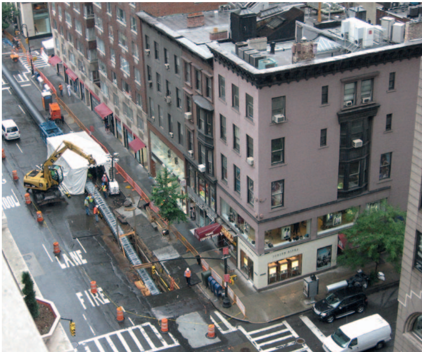
The US company Insituform completed an InsituGuard project on Madison Avenue, New York City, New York in 2009.
