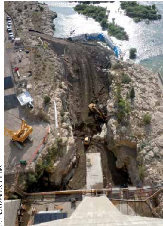
THE PUEBLO DAM CONNECTION ON THE SOUTHERN DELIVERY SYSTEM IS CONSTRUCTED.
