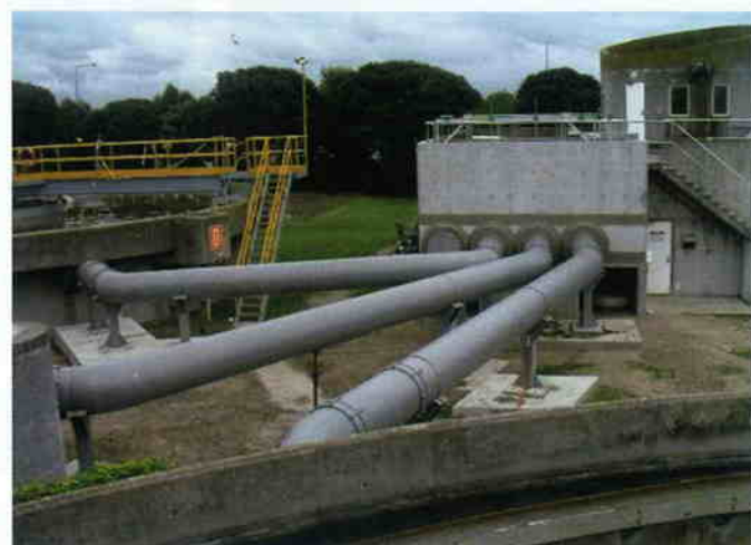
Figure 2 – New pipework to feed the primary settling tanks, and removing plant bottle-necks has increased hydraulic capacity
