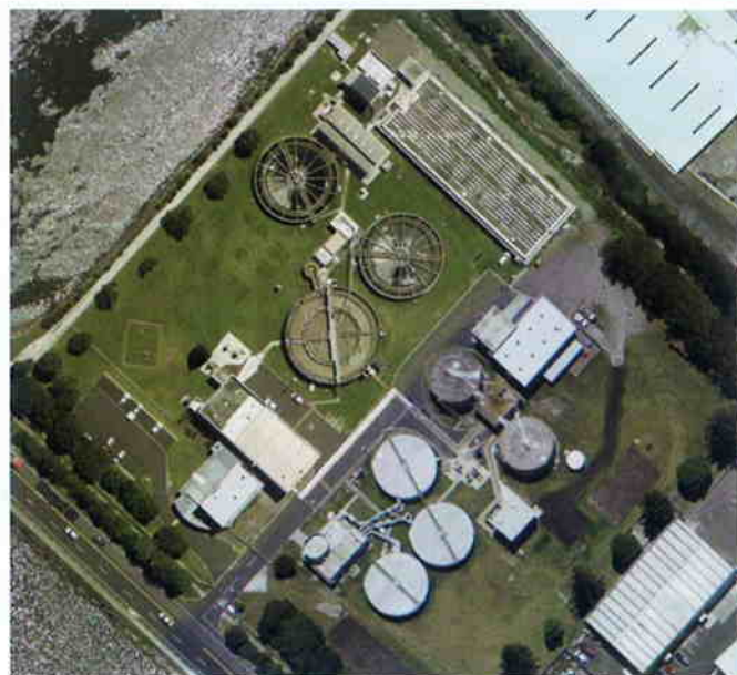
Figure 1 – Aerial view of the Chapel Street WWTP 1
