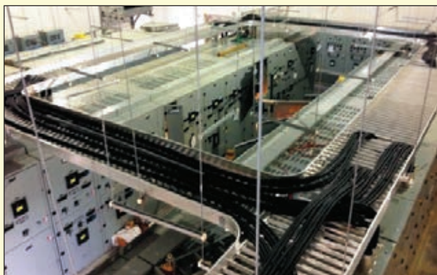
Figure 4B. View on Double-Ended Main and Generator Switchgear.
