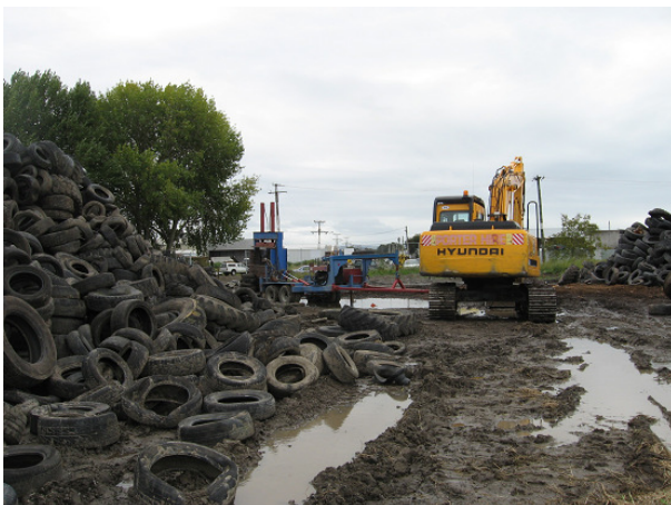
Photo 10: Ponding due to poor drainage Photo 11: Dusty site conditions in summer
