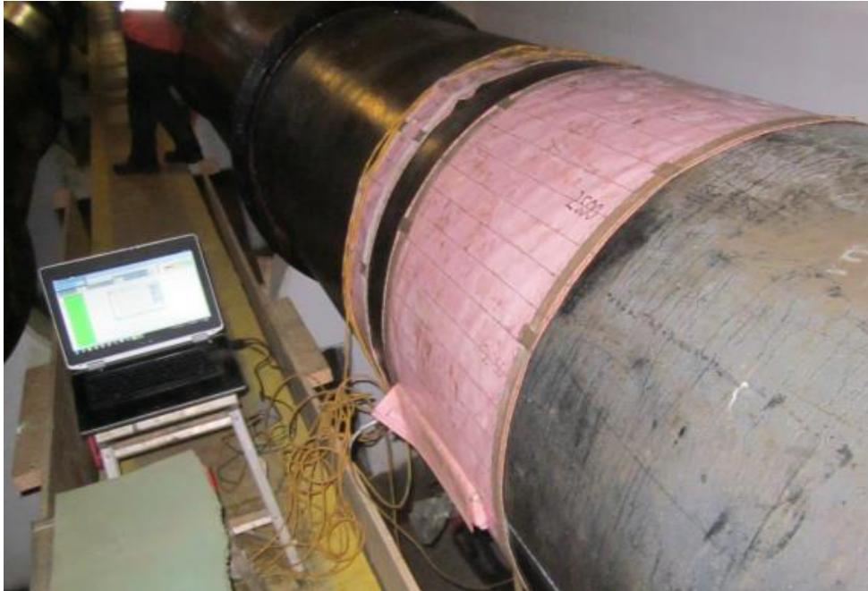
A circular saddle was wrapped around the pipe so that its thickness could be monitored using the BEM sensor equipment. Lines on the saddle every 50mm indicated where measurements were taken.
