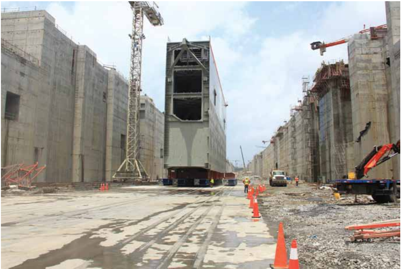
The new steel lock gates are 30m high, 58m long, between 8-10m wide and weigh up to 4,400 tons.
