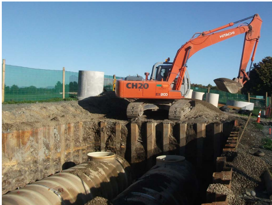
Installation of the two 30m 3 propriety fibre-glass storage chambers
