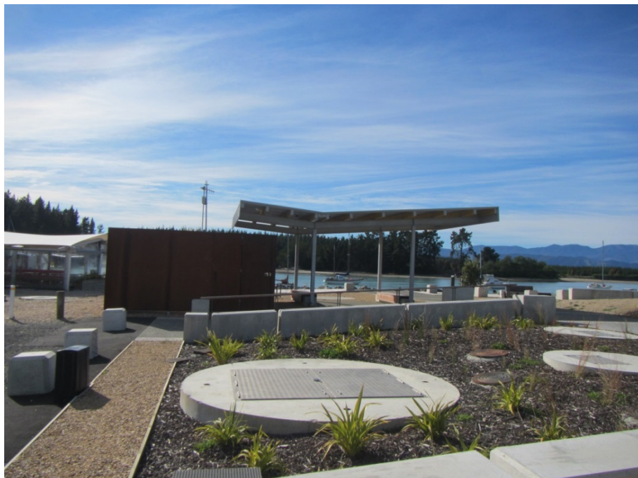
The finished product: a pump station that blends with its surroundings including the restaurant and a public recreation area
