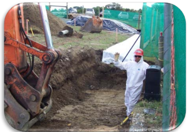
Figure 1: Staff wearing protective equipment during excavations in contaminated land
