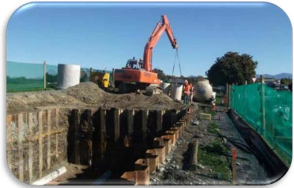
Figure 2: sheet-piling into dense, weathered Moutere gravels provided excellent groundwater cut off
