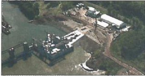
An aerial shot of the new hydroelectric facility at the Willow Island Locks and Dam in Pleasants County.
