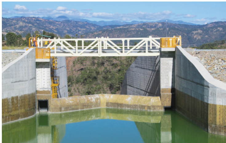
The Marlin mine spillway inlet shows the top of the spillway wall and the sluice gates for controlled discharge
