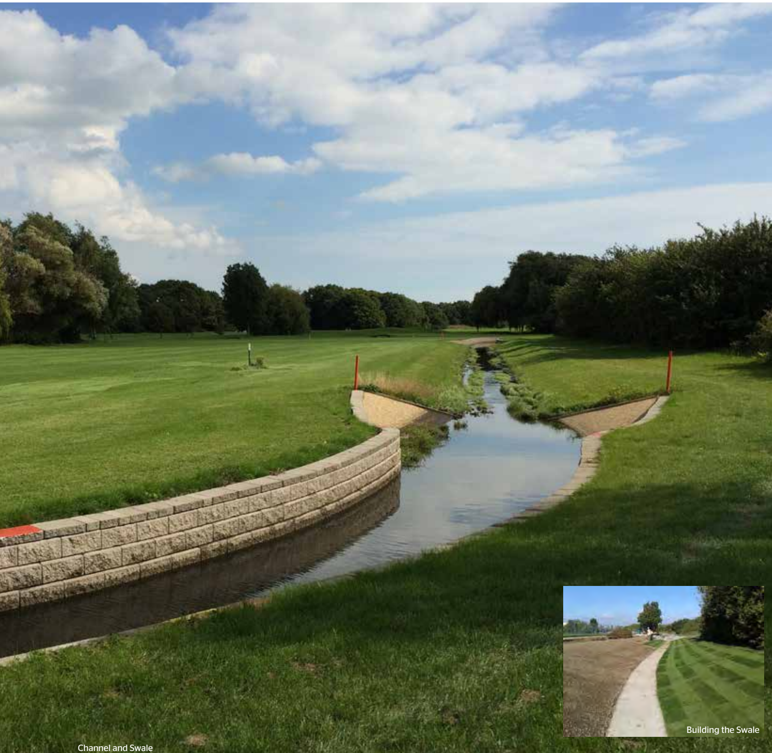
Channel and Swale
