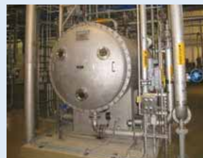
An ozone generator installed at the Shoal Creek Filter Plant. Photo courtesy of Gwinnett County Department of Water Resources
