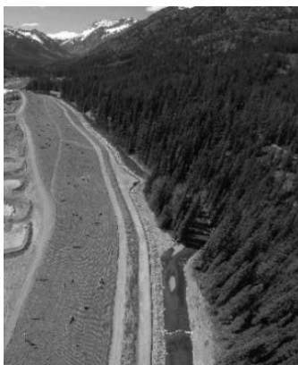
Figure 6 Photograph of restored Railroad Creek looking west up valley and regraded tailings
