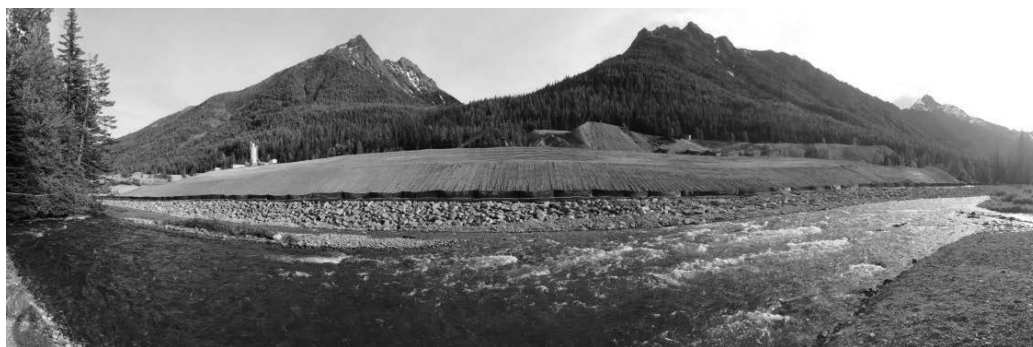
Figure 7 Photograph looking south across Railroad Creek at the south bank riprap and regraded tailings pile
