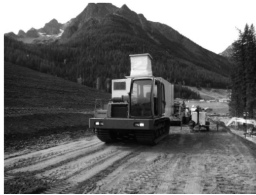
Figure 11 CPT rig on working bench in advance of jet grouting. Regraded tailings pile slope shown on left side of photo
