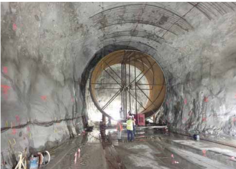
Left: Steel liner in tunnel. Photo by MWH
