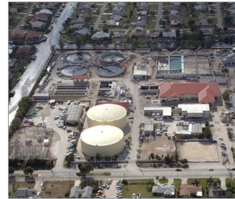
Everest Water Reclamation Facility City of Cape Coral Cape Coral, FL
