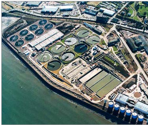
Seafeld Odor/Inlet Improvement Project Stirling Water (Seafield) Ltd Edinburgh, U.K.
