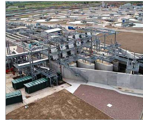
Minworth EBPR Plant Severn Trent Water Birmingham, U.K.
